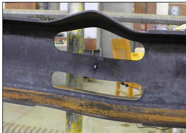
Figure 5.34 Deteriorated pile bent deteriorated section global section failure
