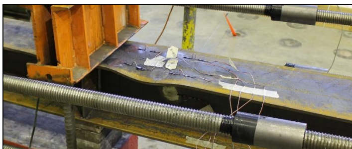
Figure 5.27 Non-deteriorated pile bent local buckling of base section
