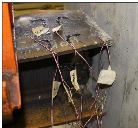
Figure 5.19 Retrofitted abutment buckling of base section
